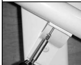
Pre-drill and insert screws from below. Repeat at all bracket locations. Check handrail
