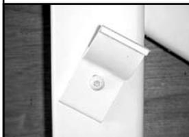
Attach handrail brackets with 3/8"-16 x 1-1/2" bolts. Do not tighten completely at this time to allow for adjustment.
