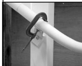
Cut and fit the 1-1/2" vinyl to follow your layout. Starting at the top of the handrail installation
