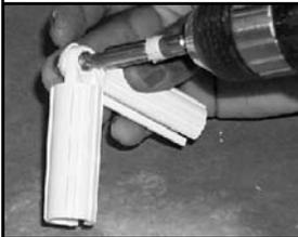
NOTE: All adjustable joiners should be supported by a handrail bracket as closely as possible to each side of the joint.
