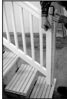
Using a level and a tape measure, lightly mark the location of the top of the handrail onto the wall or post, at the mounting position and snap a chalk line from top to bottom.
